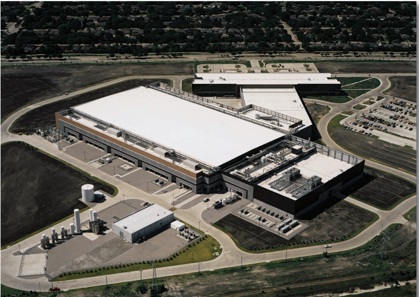
TI's new RFAB in Richardson/Texas incorporating 300mm wafer manufacturing equipment for analog and power semiconductors
