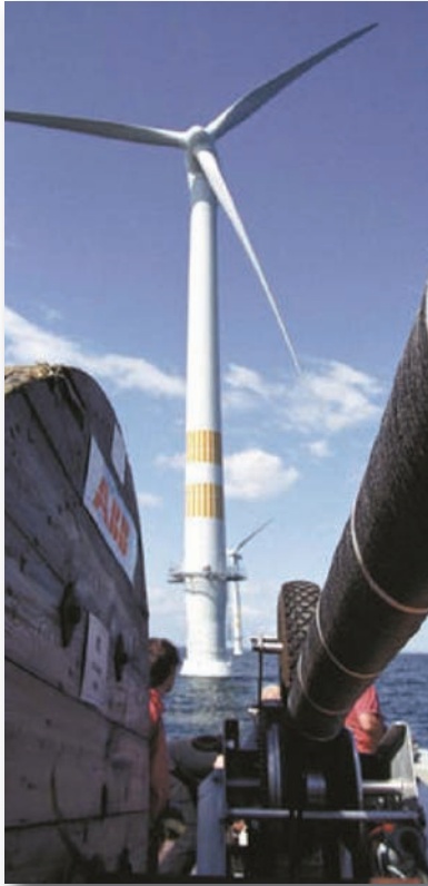
Figure 4: Sea cable for an HVDC Light™ system is laid out for connection of an off-shore wind park to the main land grid
