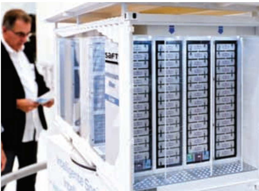
The latest trend in solar power is on-site consumption backed by battery storage systems shown at Intersolar 2013
