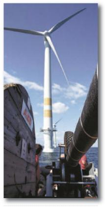
Figure 4: Sea cable for an HVDC Light<sup>™</sup> system is laid out for connection of an off-shore wind park to the main land grid
