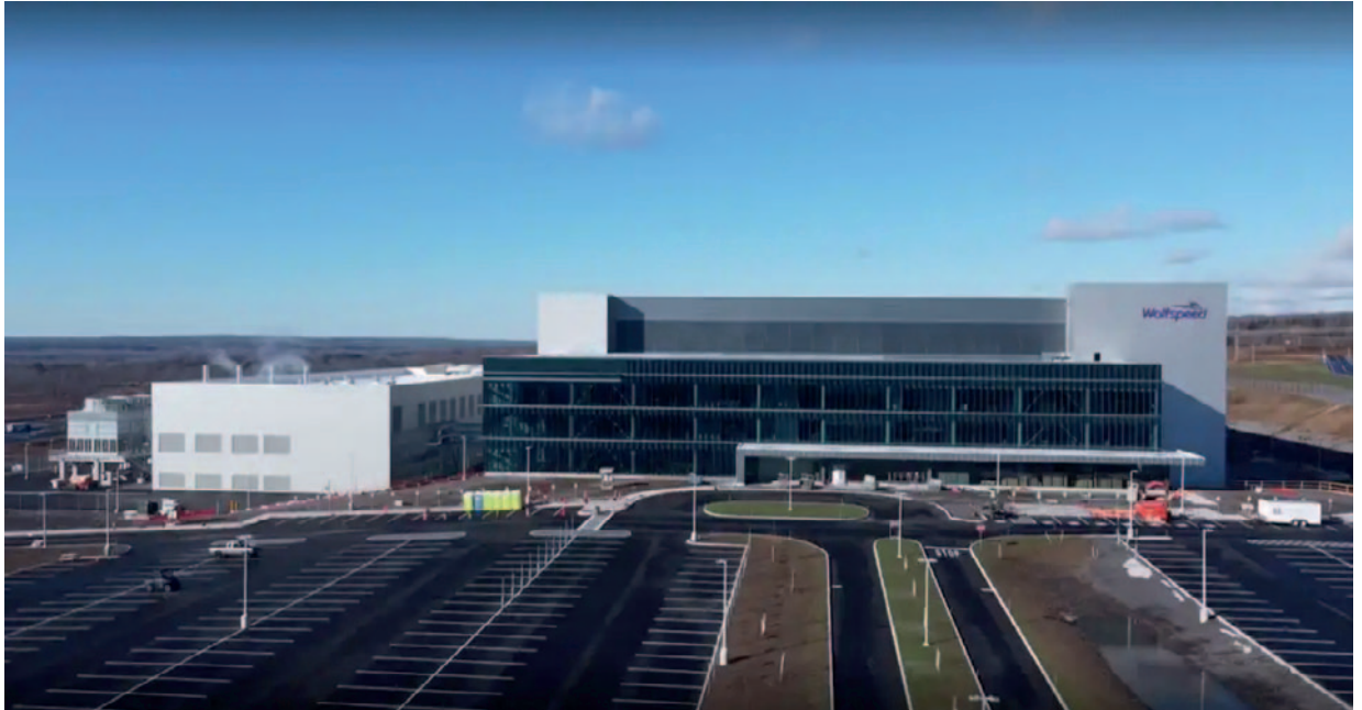
Figure 2: Wolfspeed is leading the industry in taking 200-mm Silicon Carbide wafers from prototype to production. The new Mohawk Valley Factory fabrication facility is shown above.
